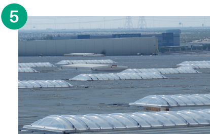
Vaulted SSR Rooflights (Standing Seam)
