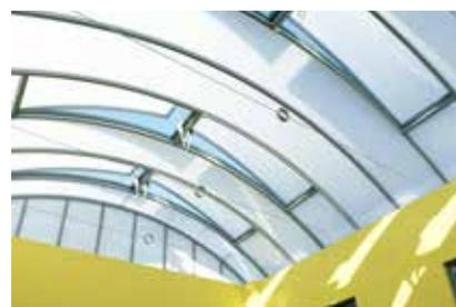
The attention to detail is evident in the clean lines and minimalist styling of the Marvault framework. Daylight area is maximised through wide bay centres.
