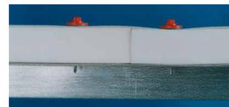
LEFT: Fixing through Hardpak rigid internal support - tightened to give an effective seal. RIGHT: Fixing through high density filler - causing 'dishing' around the fastener.
