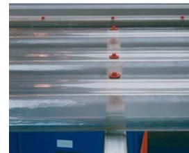
**The specification of internal supports, alignment relative to the purlin, and method of fixing are critical to achieving a good FAIR installation.**
