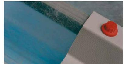
Galvanised steel strip bonded into side lap
