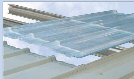
**It is essential that sufficient support is provided to the FAIR outer sheet beneath each fixing to achieve these requirements, enabling fastener washers and sealants to be compressed for a good seal whilst preventing deflection of the outer sheet.**
