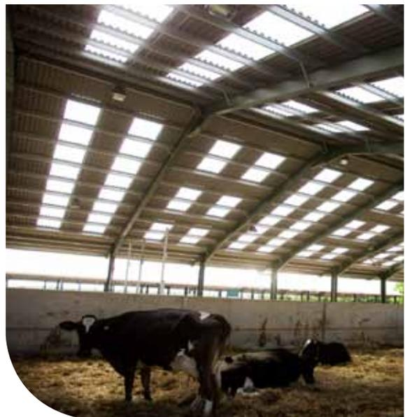
Brett Martin also manufactures polyester factory assembled triple glazed, insulating rooflights for quick and simple installation on site.
